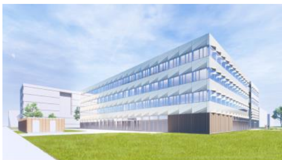
Project Next Delft
